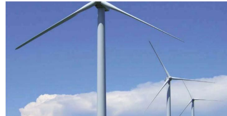
Wind turbines are available from on-shore applications in capacities ranging from 1kW to 5MW and both vertical and horizontal axis turbines are readily available. Horizontal axis turbines are the most usual form and have turbine blades spinning perpendicular to the ground with the turbine shaft horizontal to the ground. Vertical axis turbines spin horizontal to the ground with the turbine shaft perpendicular to the ground.
